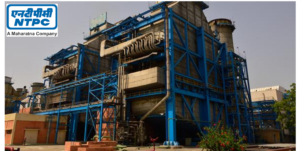
NTPC Dadri Stage II – Unit #6 490 MW
